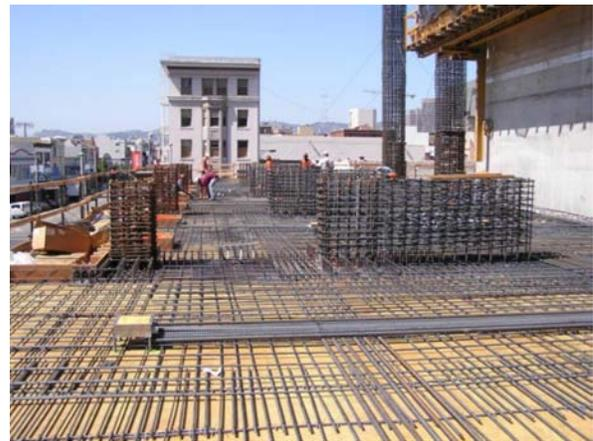
**Figure 9-6** – Conflict between the location of collector reinforcing with a nonstructural component.
