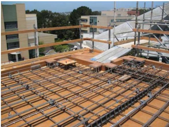
Figure 9-3 – Confinement of a collector.
