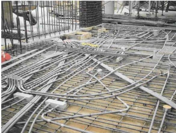
**Figure 9-5** – Embedded conduit.
