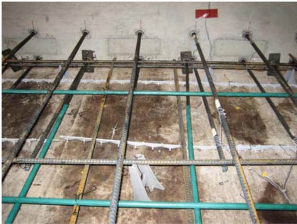
**Figure 9-4** – Form savers for dowel anchorage.
