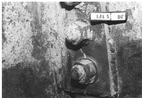
Figure 1-5 Vertical Fracture through Beam Shear Plate Connection
