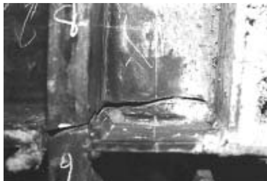
b. Fracture Progresses into Column Web
