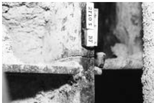
a. Fractures through Column Flange
