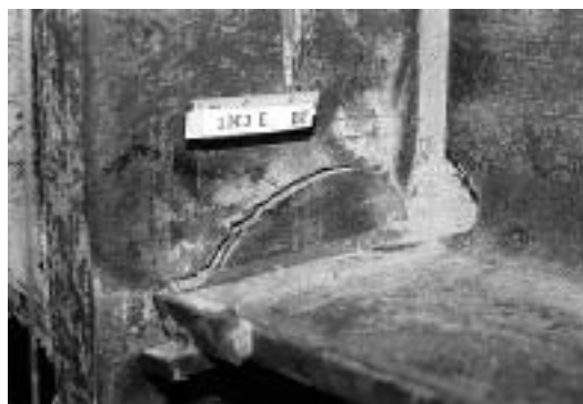
b. Column Flange "Divot" Fracture
