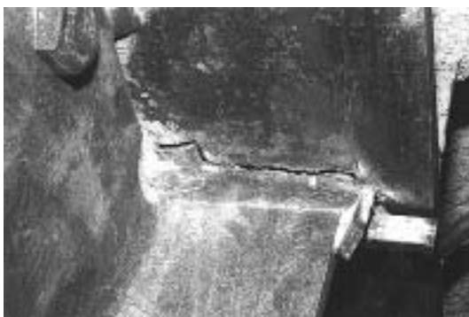
a. Fracture at Fused Zone
