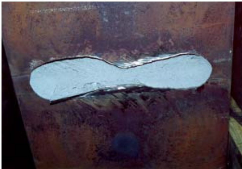
Figure 5-8 View of Divot-Type Fracture of Column Flange in Specimen with No Continuity Plates
