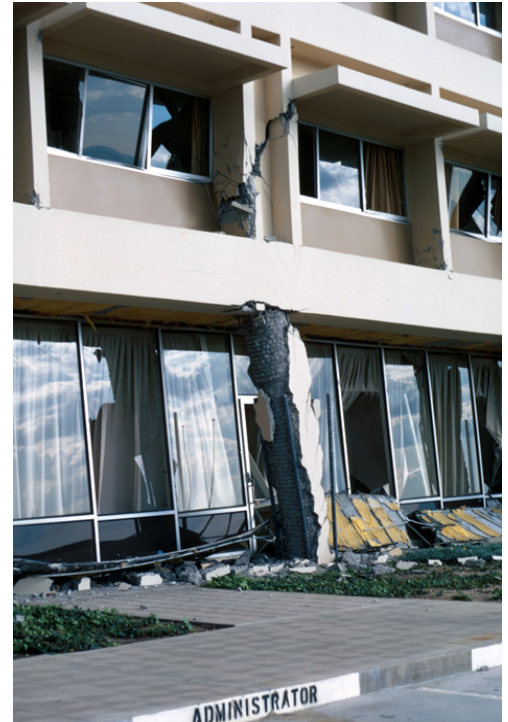
Figure 2.2 Column failure at Olive View Hospital in 1971 San Fernando earthquake (from USGS Library).
