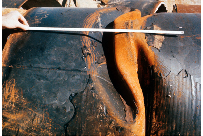
Figure 2.3 Compression failure in 49.5 inch diameter steel pipe during 1971 San Fernando earthquake (from USGS Library).
