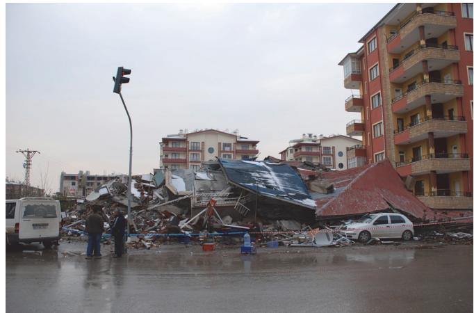
*Building collapse (38.49276N, 43.37539E) in Van, Turkey, caused by November 9, 2011, M5.6 earthquake. Structure was damaged by the October 23, 2011, M7.1 earthquake. Collapses caused by aftershocks created anxiety among the Van population and, combined with the wintry conditions, prompted a large migration of families from Van. Credit: T. Holzer, USGS.*
