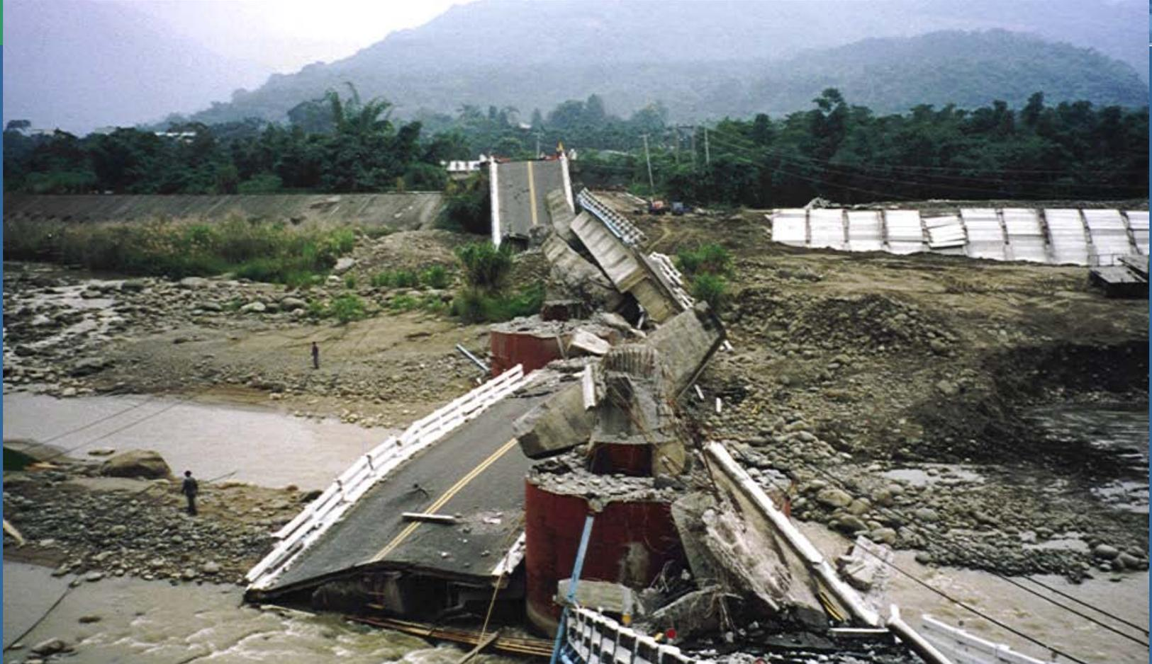
Failure of shear-critical columns in Tong-tou bridge, Chi-chi Earthquake, Taiwan, September 1999
