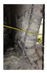
Figure 3-3 – Wall buckling, 2011 Christchurch earthquake.
