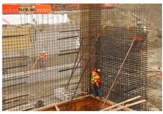
Figure 7-3 – Boundary confinement for wall flange.
