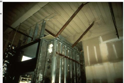
Photos and illustration from the light interior partition wall component example in FEMA E-74. Left photo (courtesy of Wiss, Janney, Elstner Associates) shows failure of inadequately braced partial height partitions in the 1994 Northridge earthquake. Center detail illustrates seismic mitigation solution for nonstructural, partial height stud wall. Photo on right (courtesy of Degenkolb Engineers) shows appropriately braced partial height stud partition.
