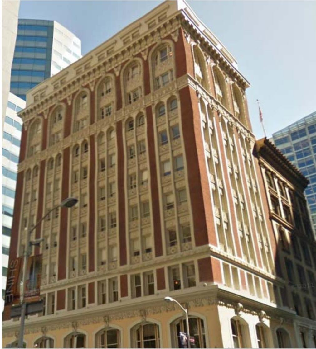
**Concrete Frames with Brick Infill**
