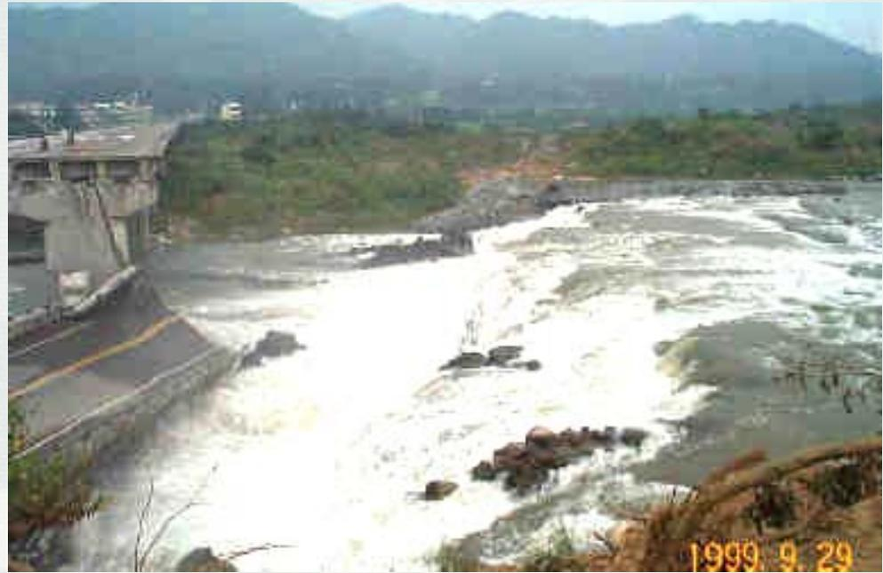
>15 ft of thrust faulting created this waterfall and destroyed bridge
